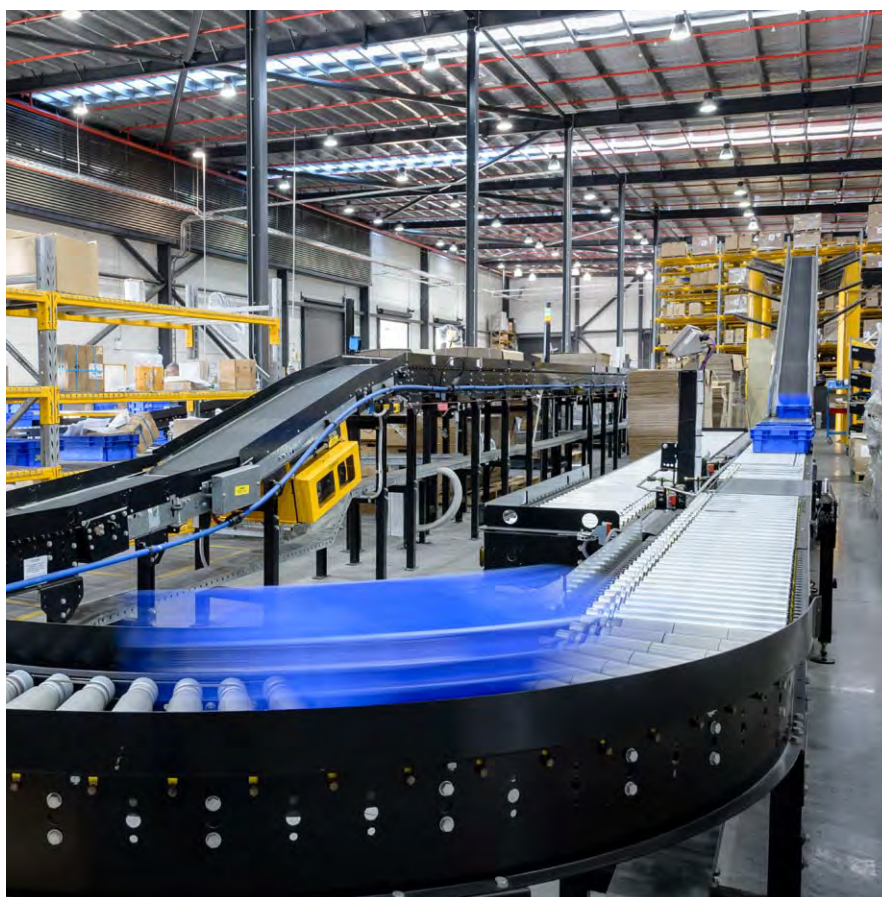
AUTOMATED WAREHOUSING SYSTEM, TOMAGO NSW
