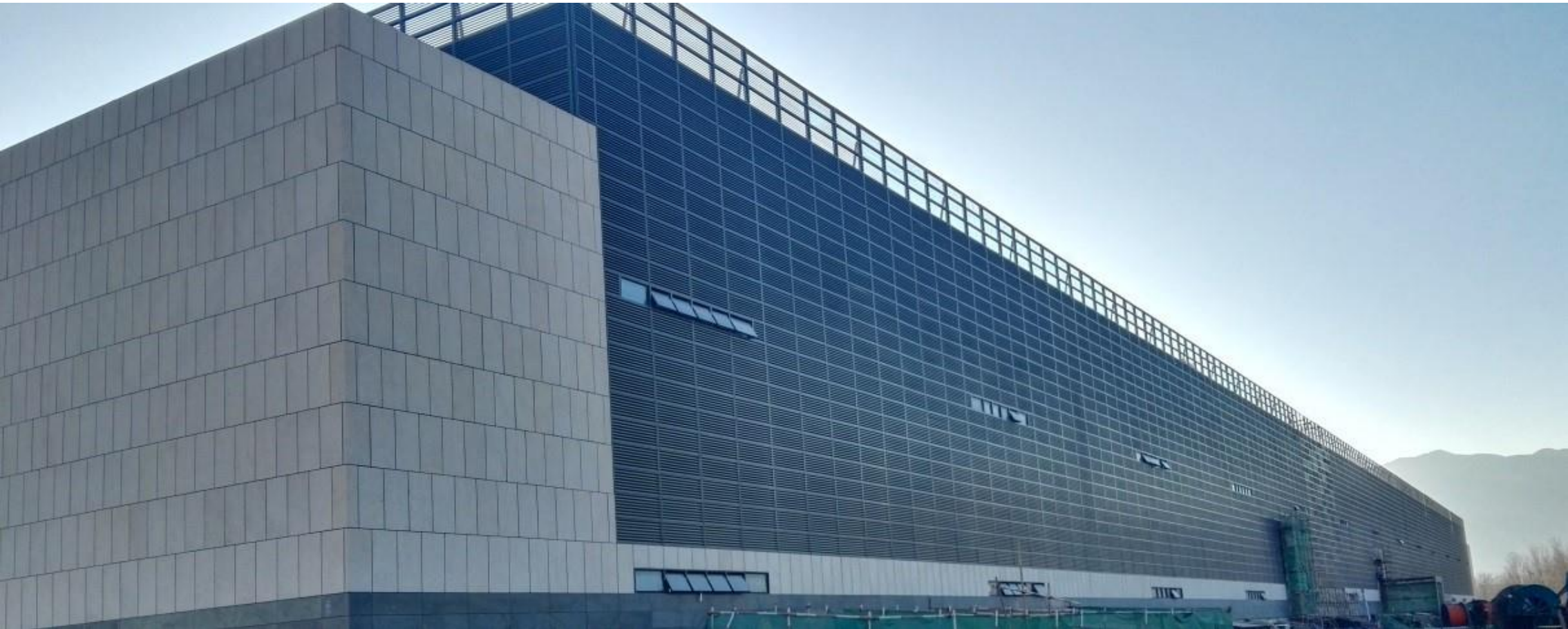
China Construction Bank's data centre relies on CAT standby generators supplied by WesTrac China
