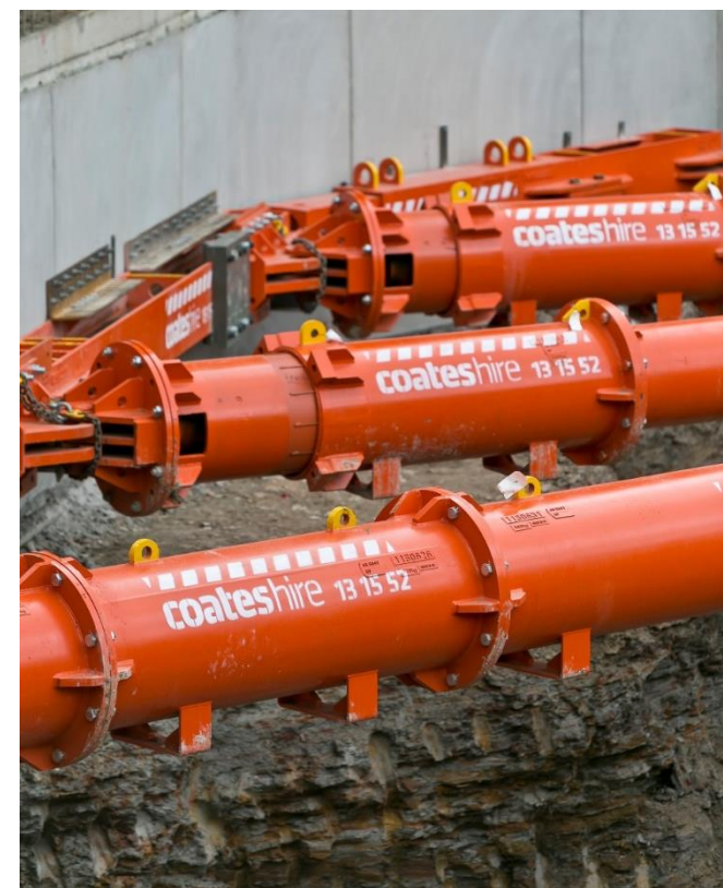
Coates Hire | Hydraulic Shoring | Sydney
