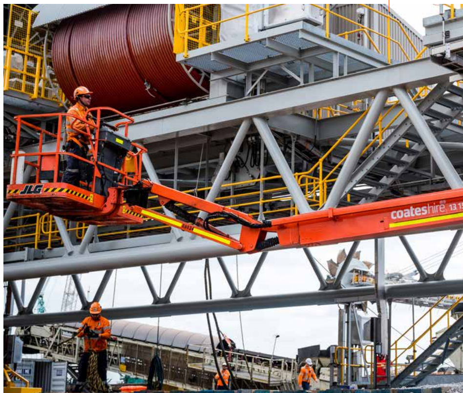
80 foot articulated boom at Port Kembla Coal Terminal.
